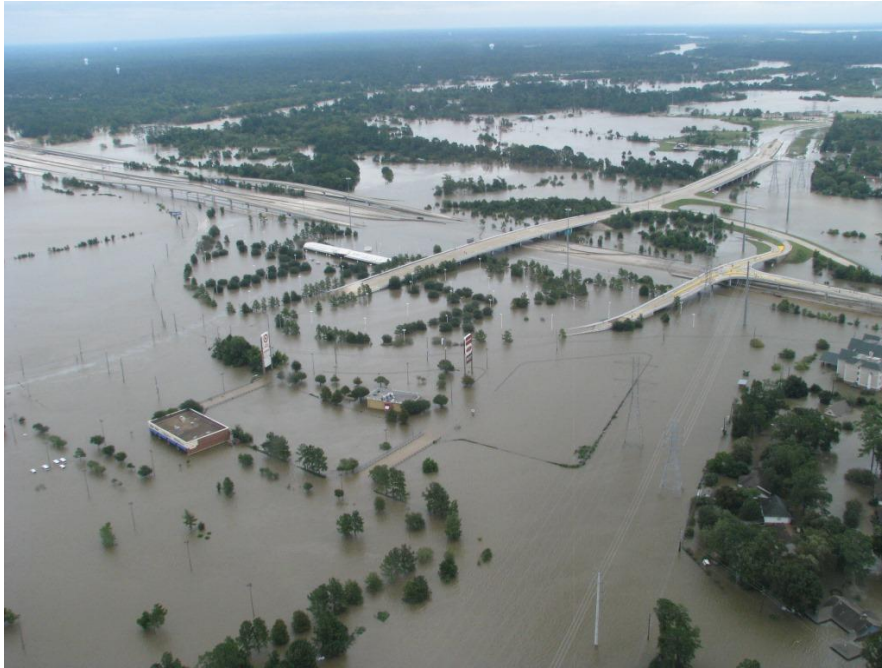
West Fork San Jacinto River near Humble, Texas after Hurricane Harvey Image: Steve Fitzgerald, Harris County Flood Control District
